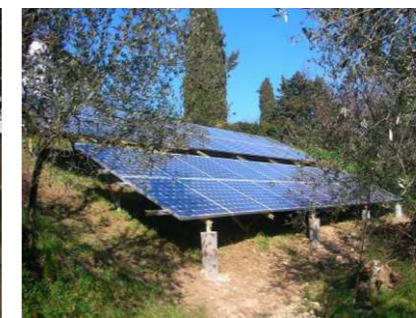
5kW project in Arezzo city, Italy, XPI-7.0kVA
