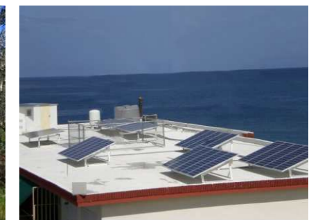
2kW project in Klang city, Malaysia, XPI-3.0kVA
