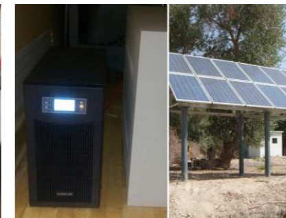
7kW Off-grid project
