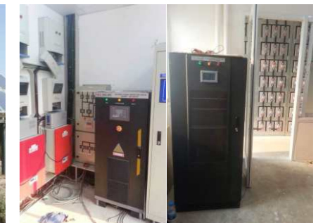
60kW project in Thailand, ETS60K
