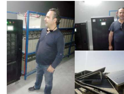
30kW Villa project in Middle East, ETS 30KVA/HSC 350M4
